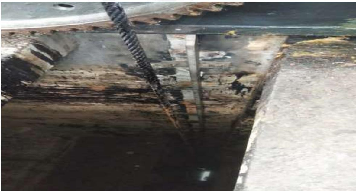
**Fig 6.4 Emergency gate guide after replacement**
