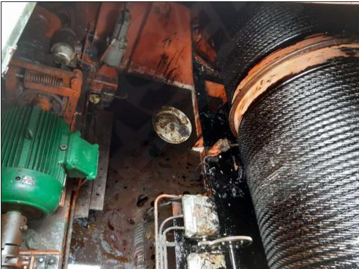
Fig 2.26 Wire rope and motor in intake gate hoist chamber
