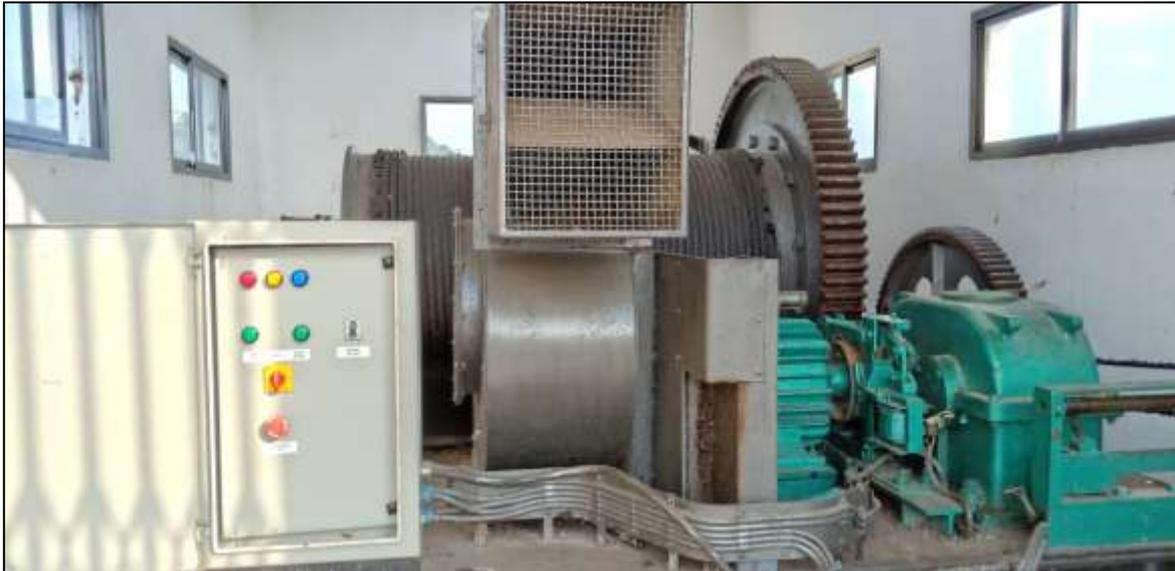
Fig 2.15 Rope drum of Emergency gate
