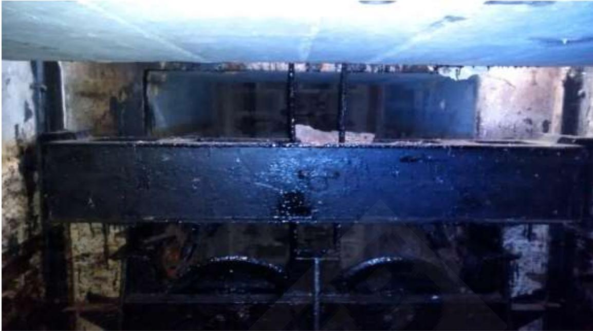
**Fig 6.3 Emergency gate guides before replacement**
