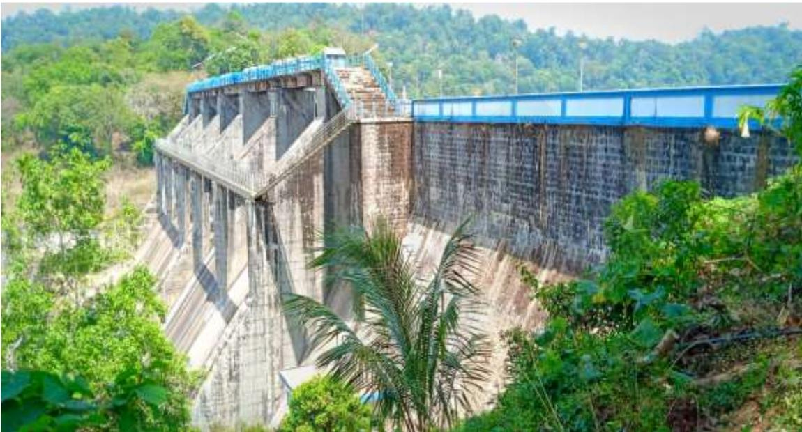
**Fig 2.4 Spillway of Sholayar Flanking Dam**
