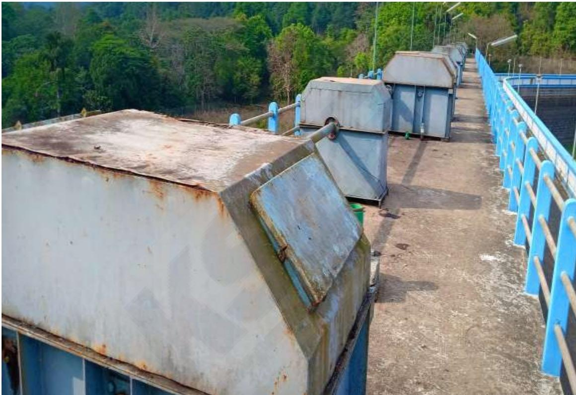
**Fig 2.5 Radial gate Hoists**
