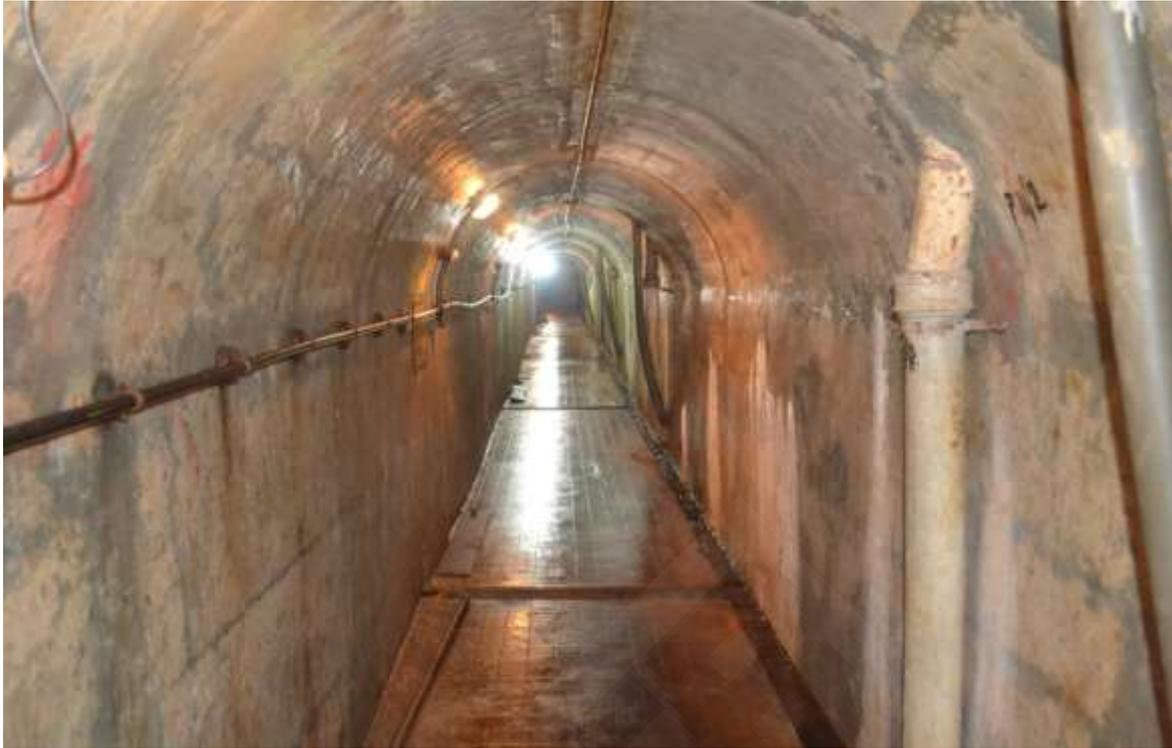
**Fig 2.9 Drainage and inspection gallery**
