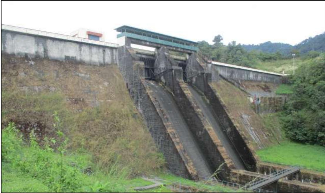
Fig 6.3 G I sheet roofing for spillway gate controlling platform
