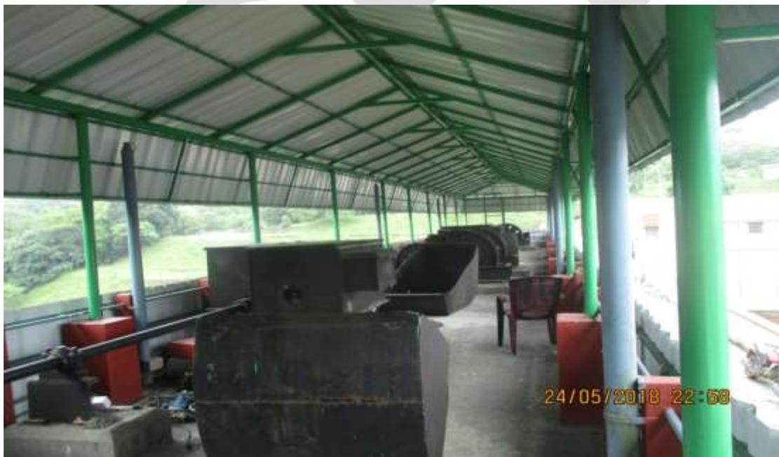
Fig 6.4 G I sheet roofing for spillway gate controlling platform
