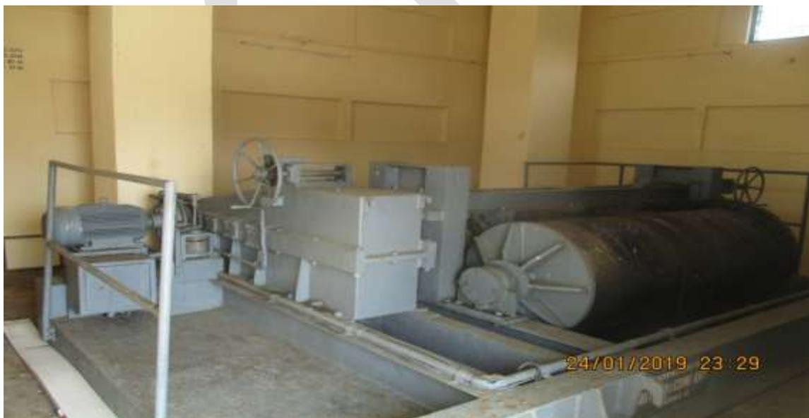
Fig 2.9 Scour gate hoisting system
