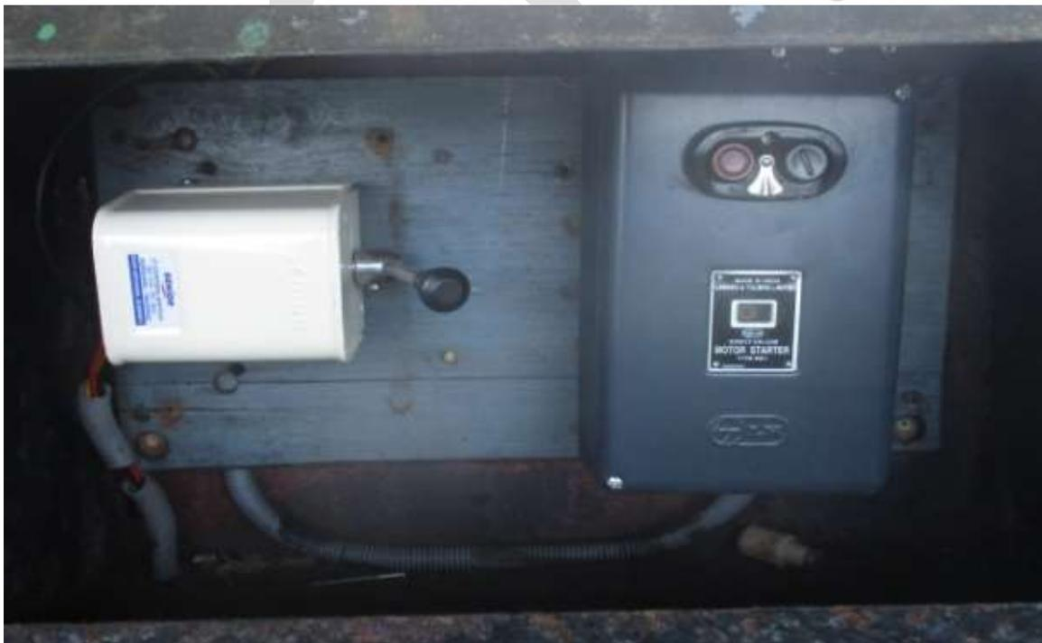
Fig 2.5 Reverse/Forward switch and starter/stopper
