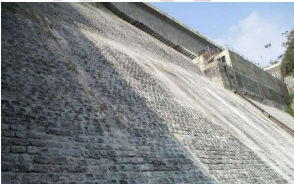
**Fig 6.6 Downstream face of dam after pressure washing and pointing**
