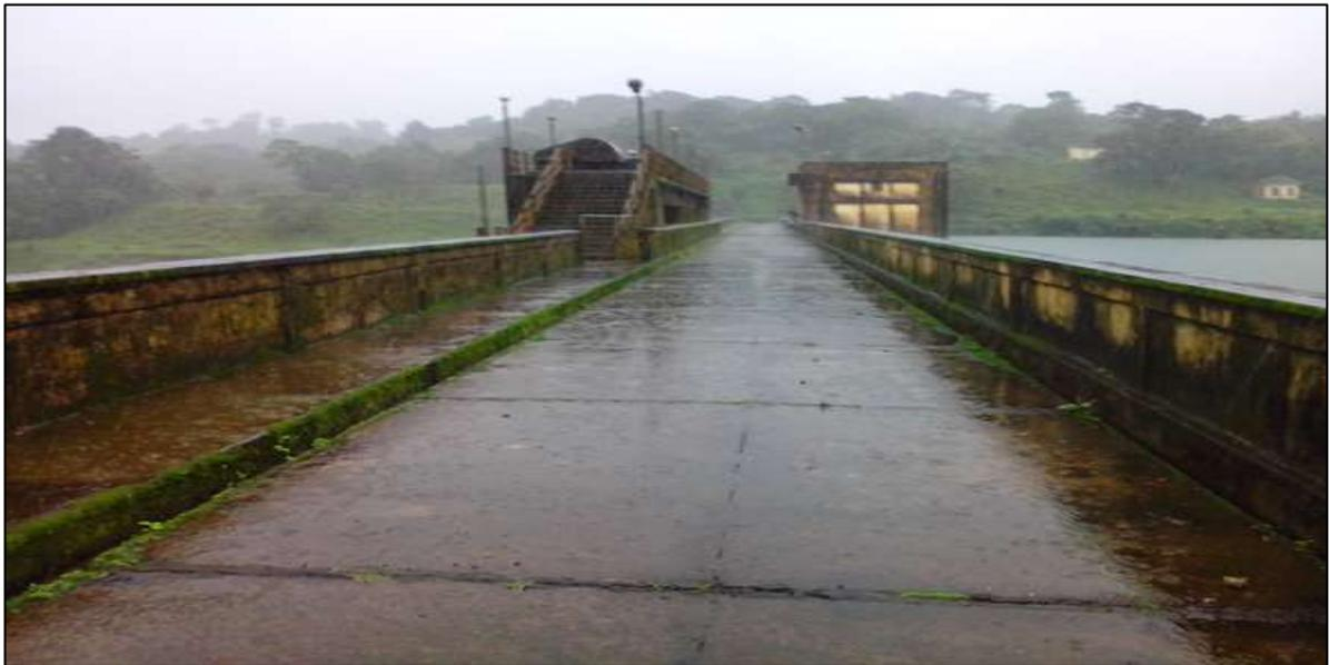
Fig 6.1 Dam top road before providing wearing coat
